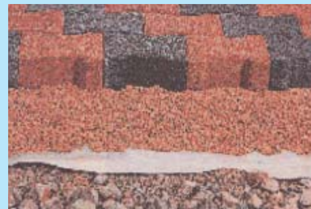
Porous Paving Details.
